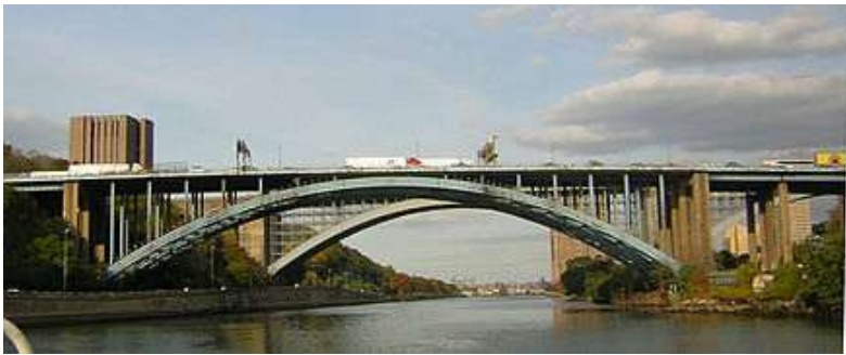
ALEXANDER HAMILTON BRIDGE-NYC
