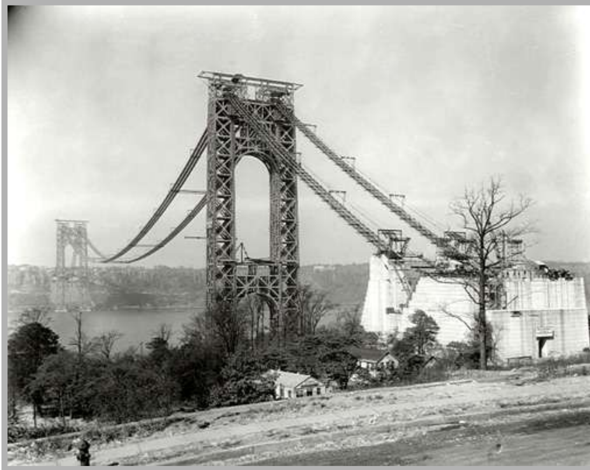
Cable Construction View From New York Anchorage Main Span - 3,500 Feet, - Longest when built Approach Spans - New York 650 Feet - New Jersey 610 Feet
